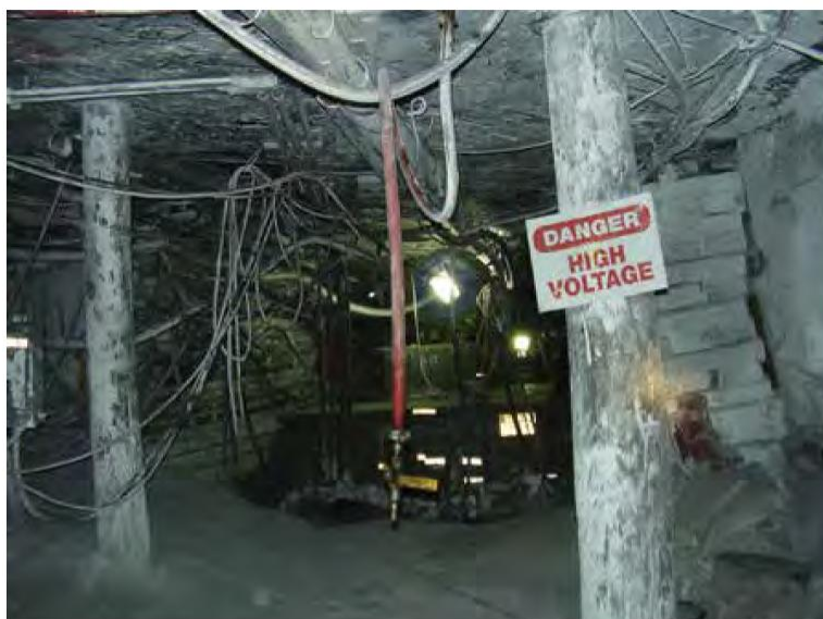
Underground at the bottom area of JWR Mine No. 4, where the coal was hoisted out of the mine. Roy Mullenix worked near here, kept the area clean, and put out rock dust to cover the black float dust, circa 2006 (Courtesy of Kristina Mullenix)
