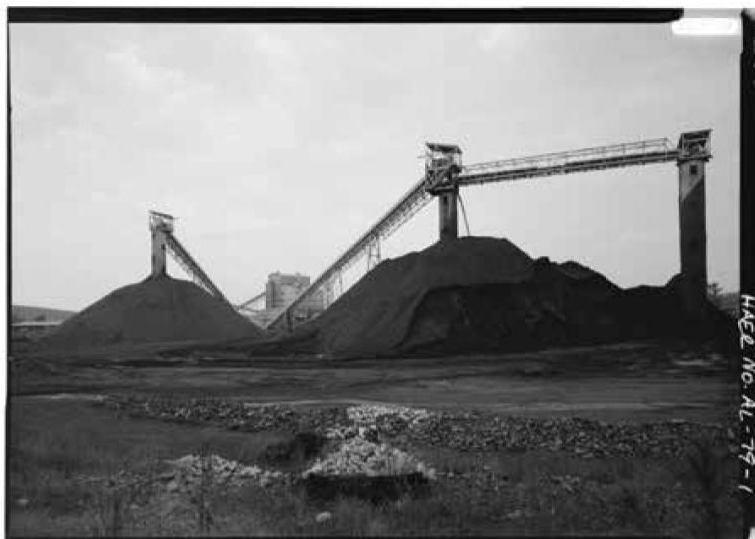
Jim Walter Resources, No. 5 Coal Mine, Lock 17 Road in Brookwood, AL (Courtesy of Library of Congress, N.D.)
